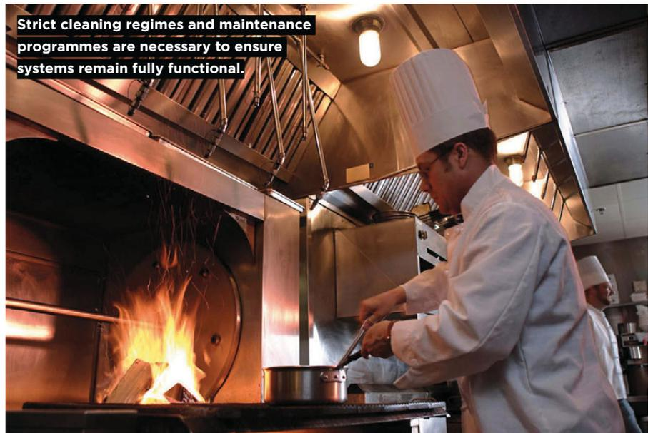
causes of commercial kitchen fires include cooking appliances being left unattended during operation, self-ignition of overheated oils, malfunctioning appliance safety switches and thermostats, fan-motor failure and grease deposits in ventilation systems.
